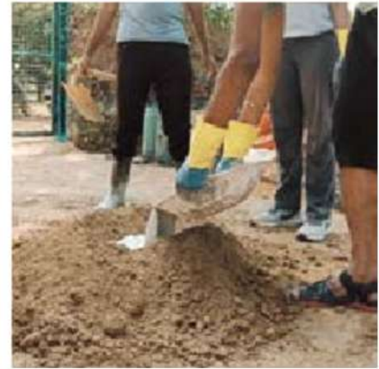
Mixing with lime
