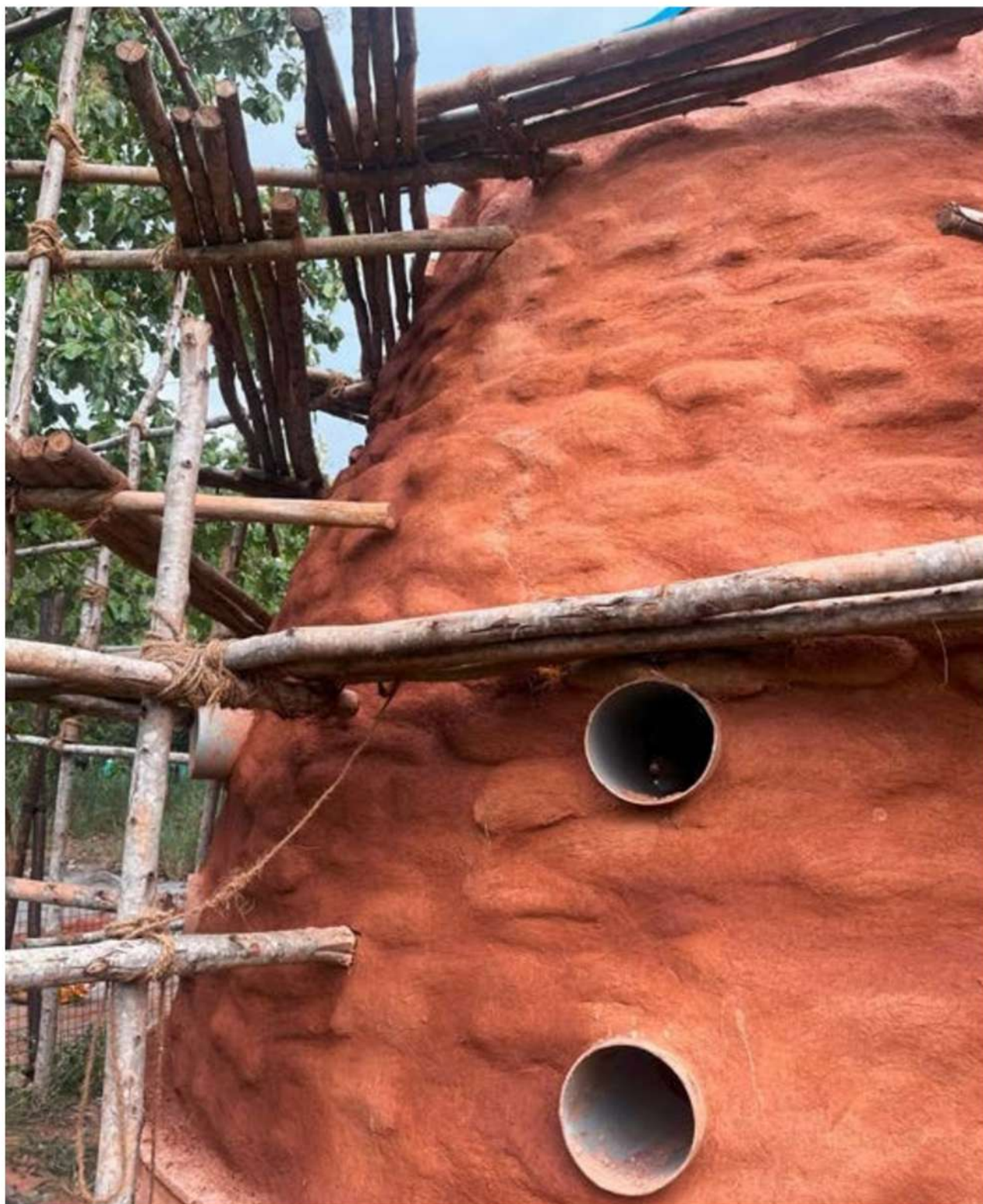
Completed earthbag dome with walls finished and plastered.
