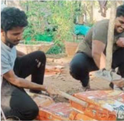
Ramming the earth bags
