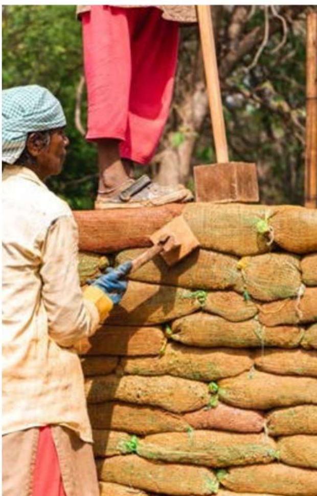
Ramming the course of bags with a wooden rammer
