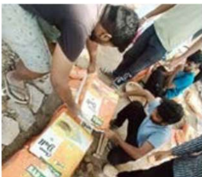
Laying of second course
