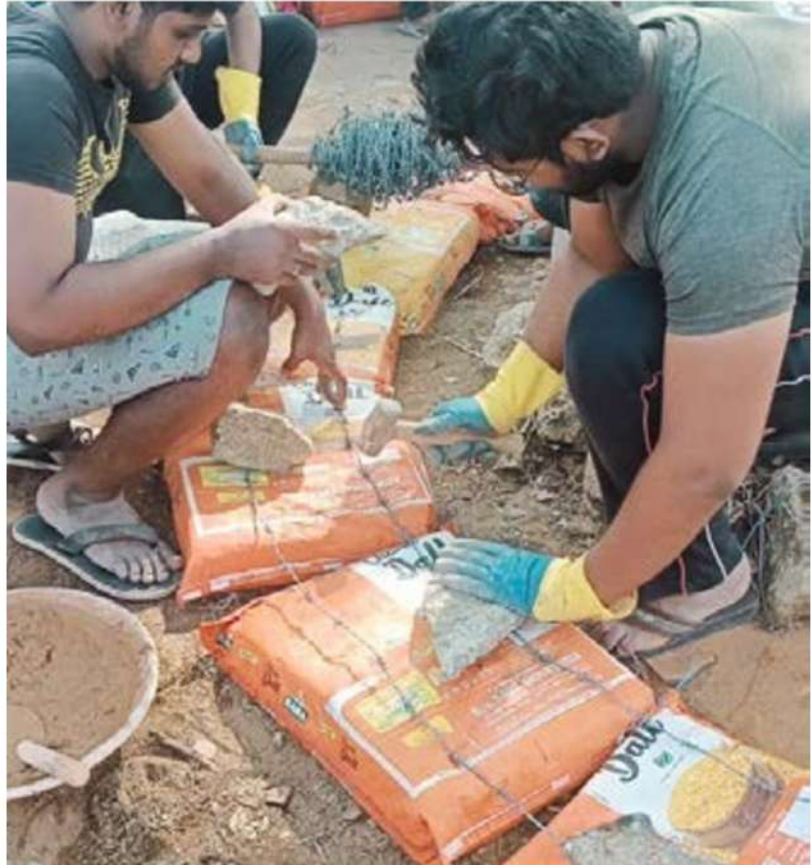
Laying of barbed wires
