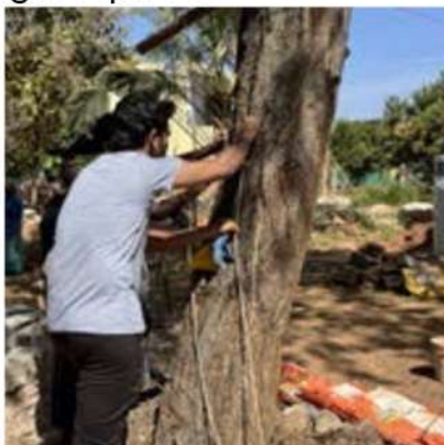
Checking of levels
