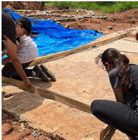
Aligning of formwork
