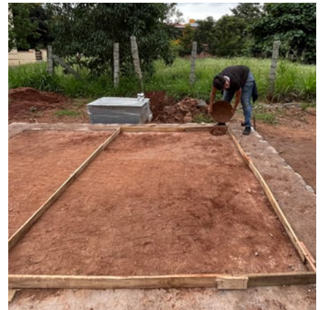
Finished formwork
