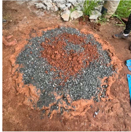
Adding and mixing surkhi and fine aggregate in small batches
