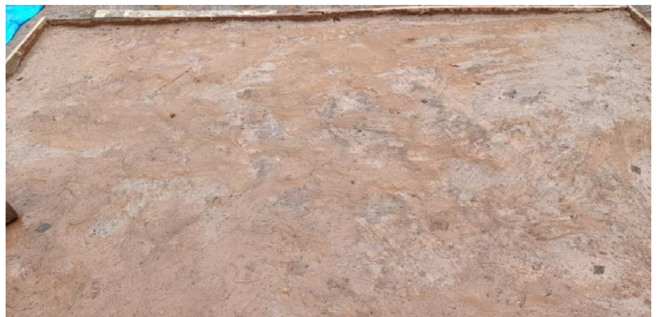
Dried surface of mud flooring
