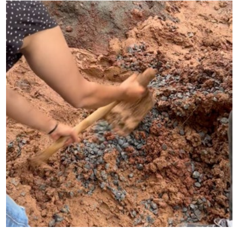
Adding and mixing surkhi and fine aggregate in small batches
