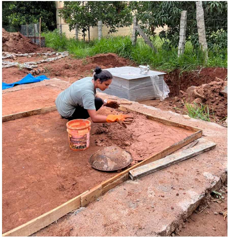
Application and spreading of the mix
