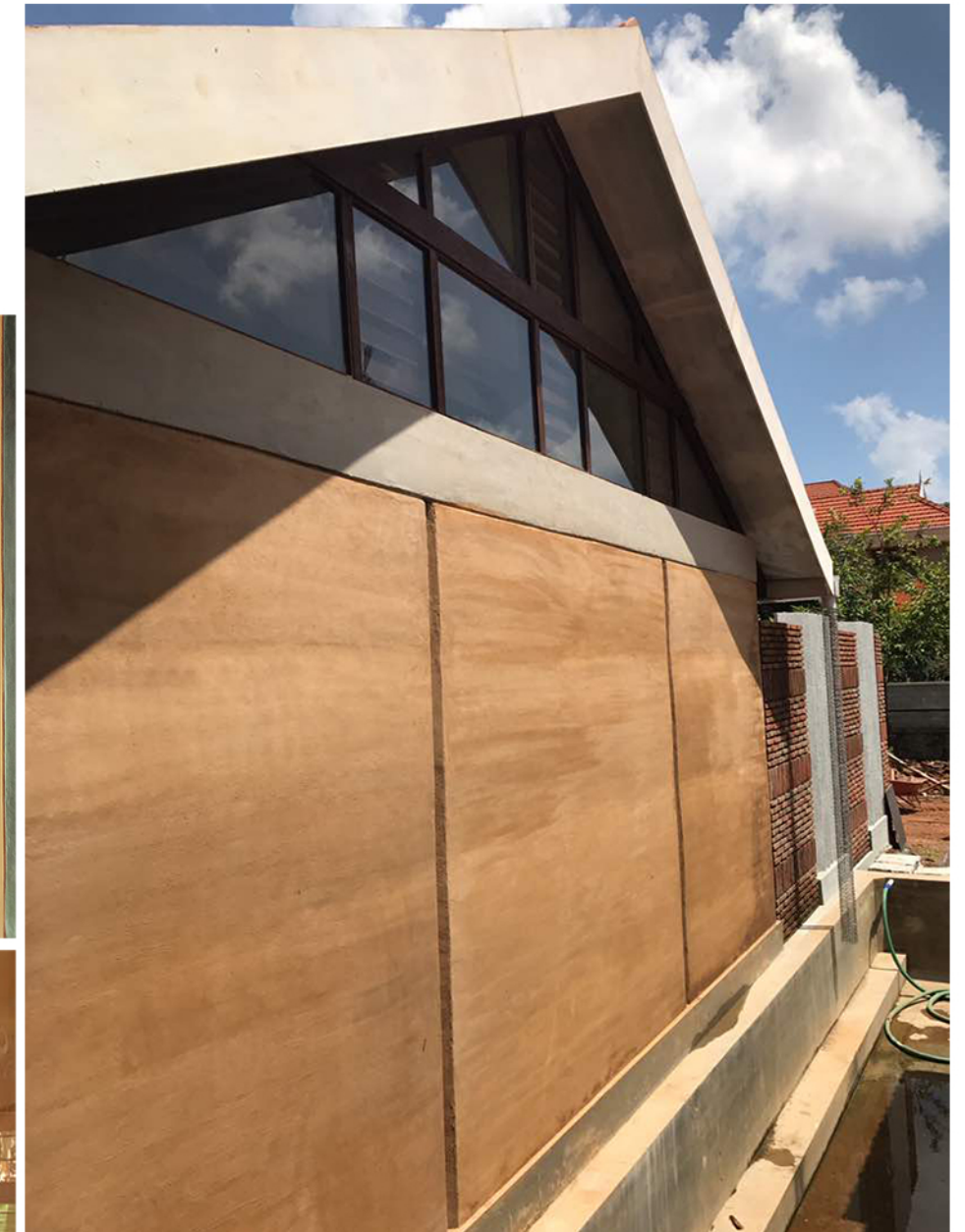
Clockwise from far left: Front view showing seminar hall entrance and brick facade of the courtyard; Verandah to the artist's studio; External rammed earth facade of the reception; Interior view of the management consultant's office; Vaulted earth roof of the seminar hall.
