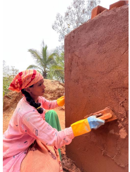
Using a Wooden Floater to smoothen the surface
