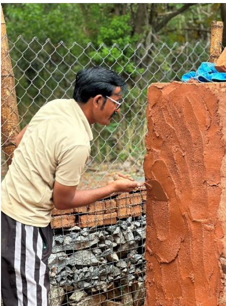
Applying Thappi plaster using a trowel
