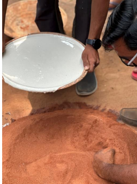
Adding Lime to Surkhi mixture
