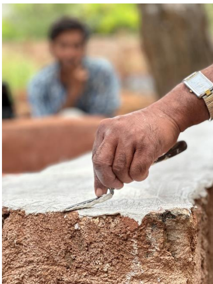
Applying a thin layer of the paste over the surface using a small trowel and levelling it with hand and trowel
