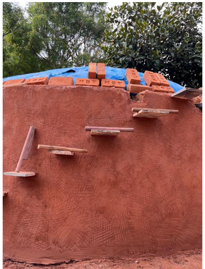
Thappi Plaster on The Hobbit House water tank
