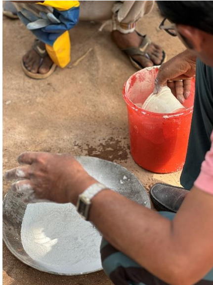
Adding Lime water to the marble dust and lime mixture
