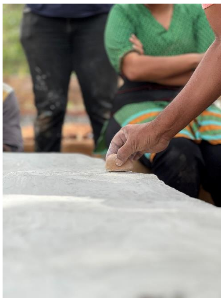
Burnishing the surface using stone
