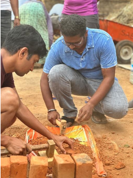
Breaking Brick into Surkhi
