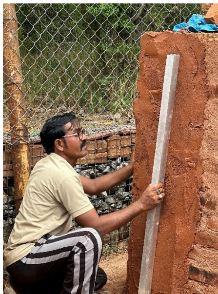
Levelling the surface using an aluminium channel
