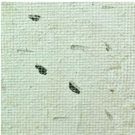
Mesh stuck to the wall
