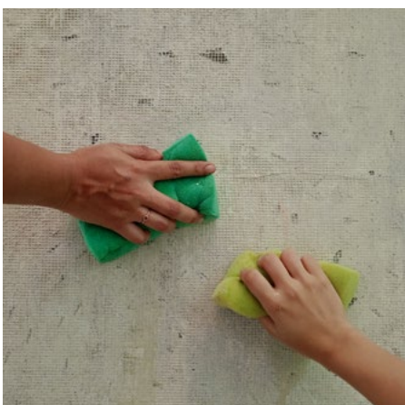
Dampening the wall
