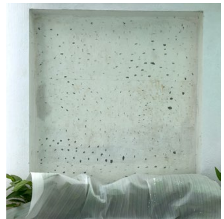
Prepared wall for base coat
