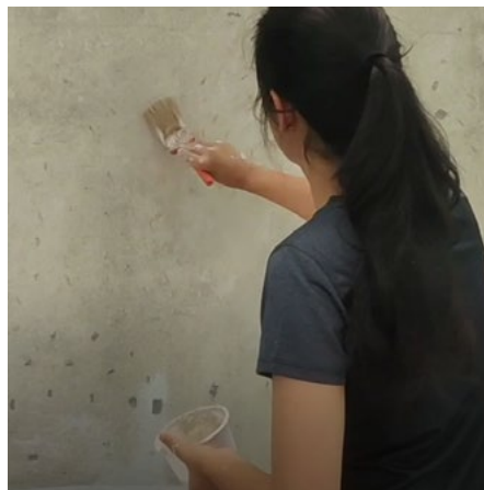
Application of lime water film
