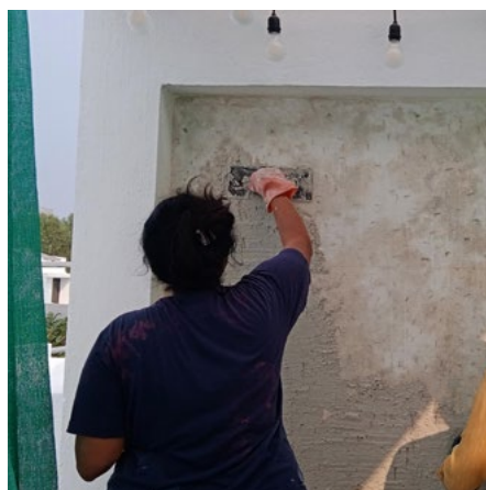
Application of base coat
