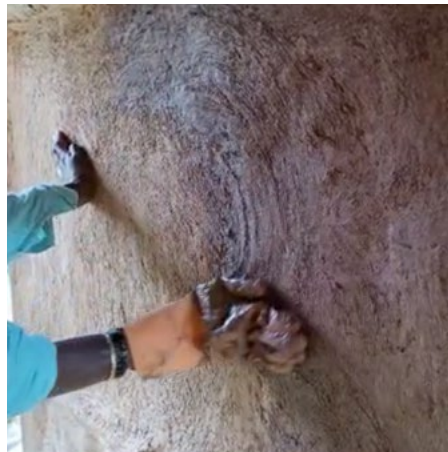
Applying the plaster
