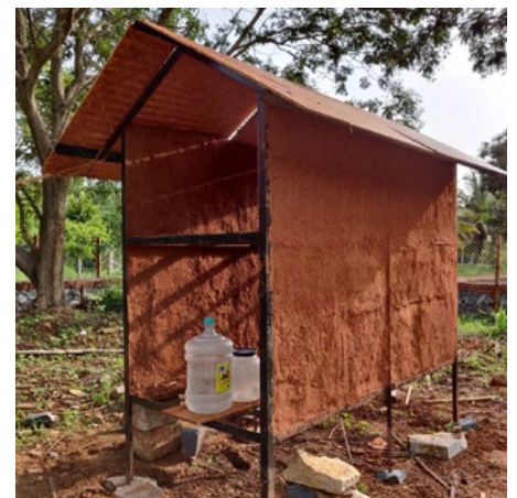
Finished wattle and daub walls
