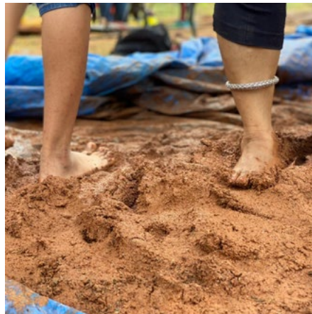
Wet mixing by stomping
