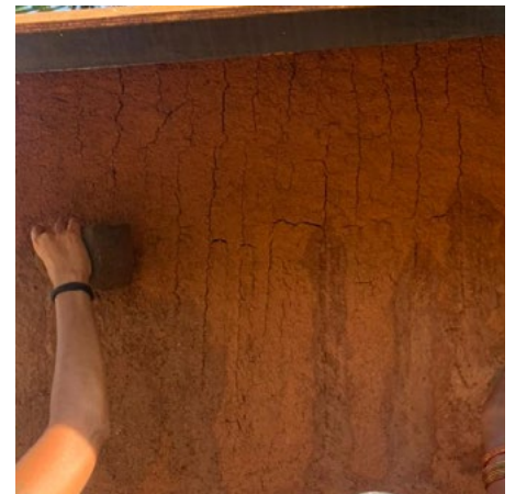
Sealing of hairline cracks
