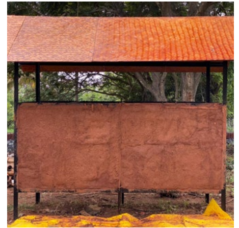
Finished wall of daub
