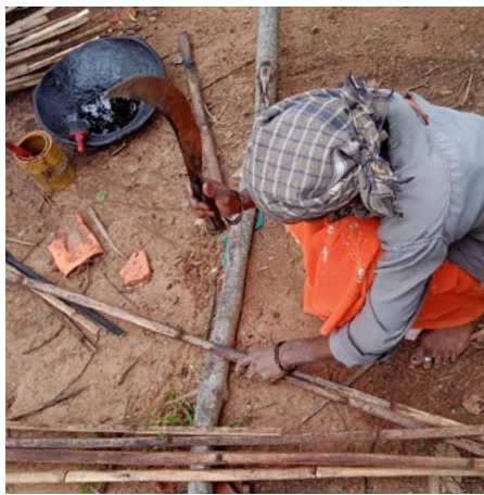
Cutting of bamboo slats to size
